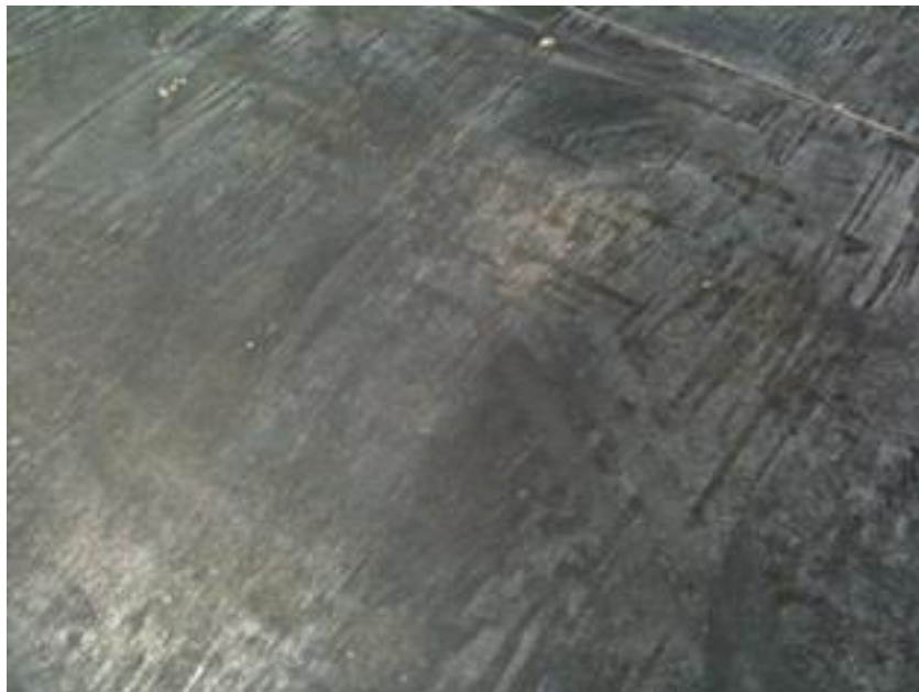
PLATE THREE: Grain Raising of the surface veneer due to weather exposure
