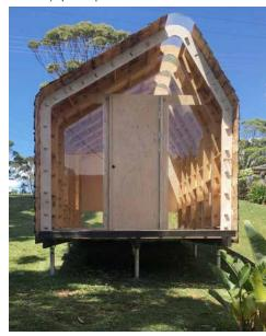
'We love the stuff. Ecoply is strong, versatile and easy to work with. Its thickness is consistent and suitable for CNC milling, ensuring all parts are structurally sound. When we went through the process of designing each part and how they might 'nest' on a standard 1200 x 2400 mm sheet of plywood, we worked painstakingly to ensure we had minimal wastage of material. This was in line with our design objective to develop a carbon neutral building kit,' said Pupilli.
