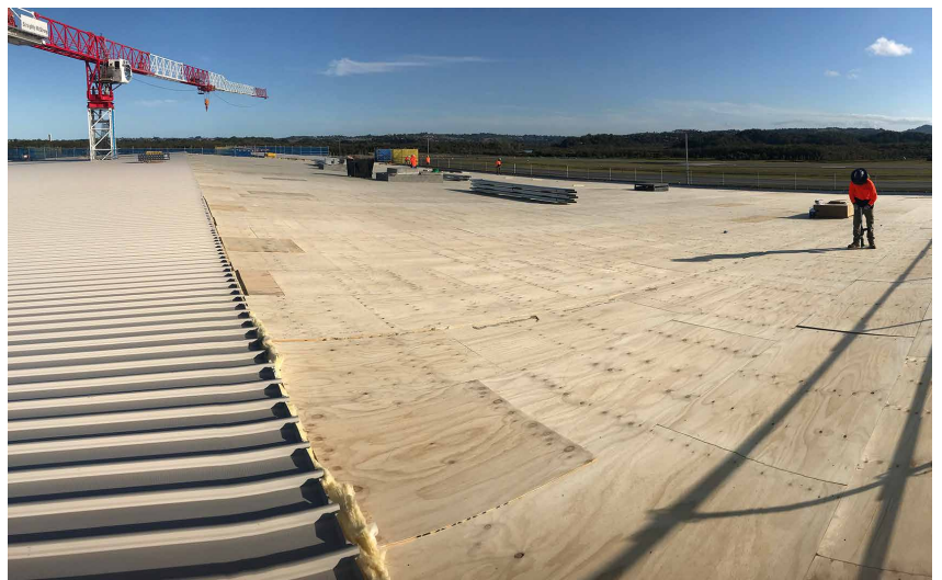
Top: Aerial photograph at Gold Coast Airport showing the terminal footprint. Photo courtesy Queensland Airports Limited. Inset: Ecoply structural plywood provides acoustic performance at Gold Coast Airport.
